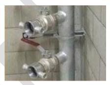
Figure 5: Typical charged riser outlet
