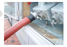
Figure 8: Insufficient clearance, hose rubs on bottom edge
