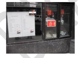
Figure 7: Clear space, sloping splash guard to base
