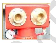
Figure 4: Two-way charged riser inlet
