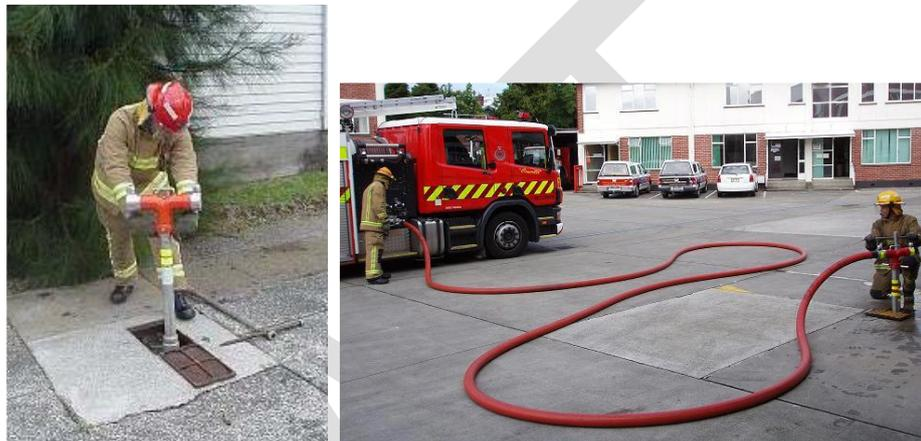
Figure 1: Typical in ground fire hydrant
