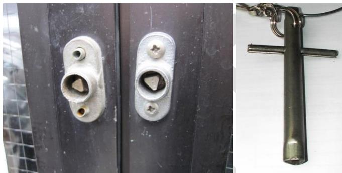
Figure 2: Fire sprinkler inlet enclosure locking device and key
