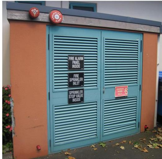
Figure 1: Fire sprinkler inlet enclosure
