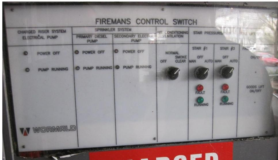
Figure 2: Photo showing basic fan controls incorporated in a panel
