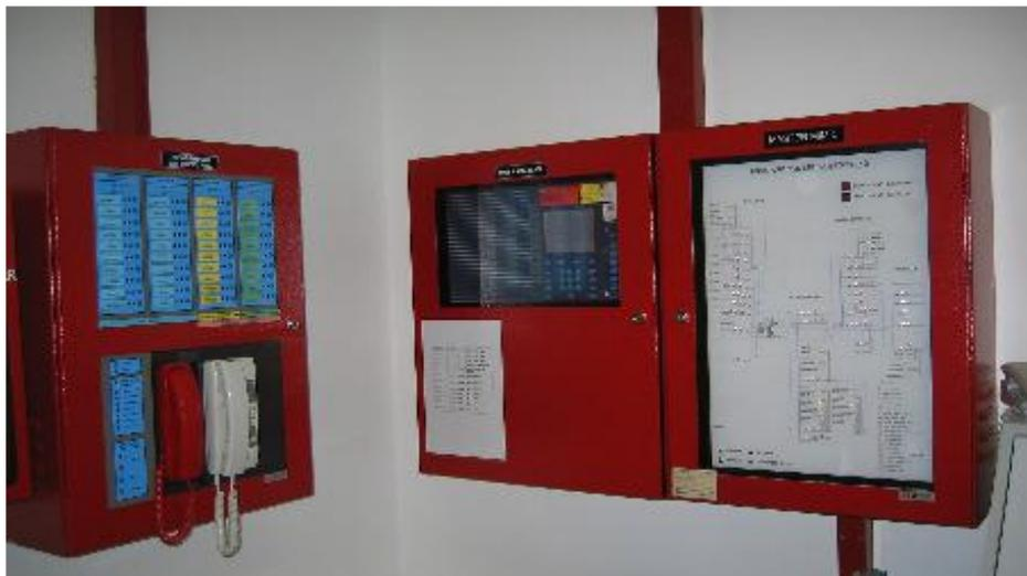
**Figure 9: Some of the equipment found in a typical fire control centre**
