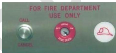
Figure 4: Typical key panel in fire service elevator cab
