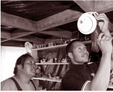
More than 12,000 smoke alarms were installed in Northland homes
