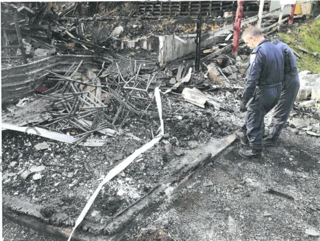
Photo 10 showing storeroom during early excavation.
