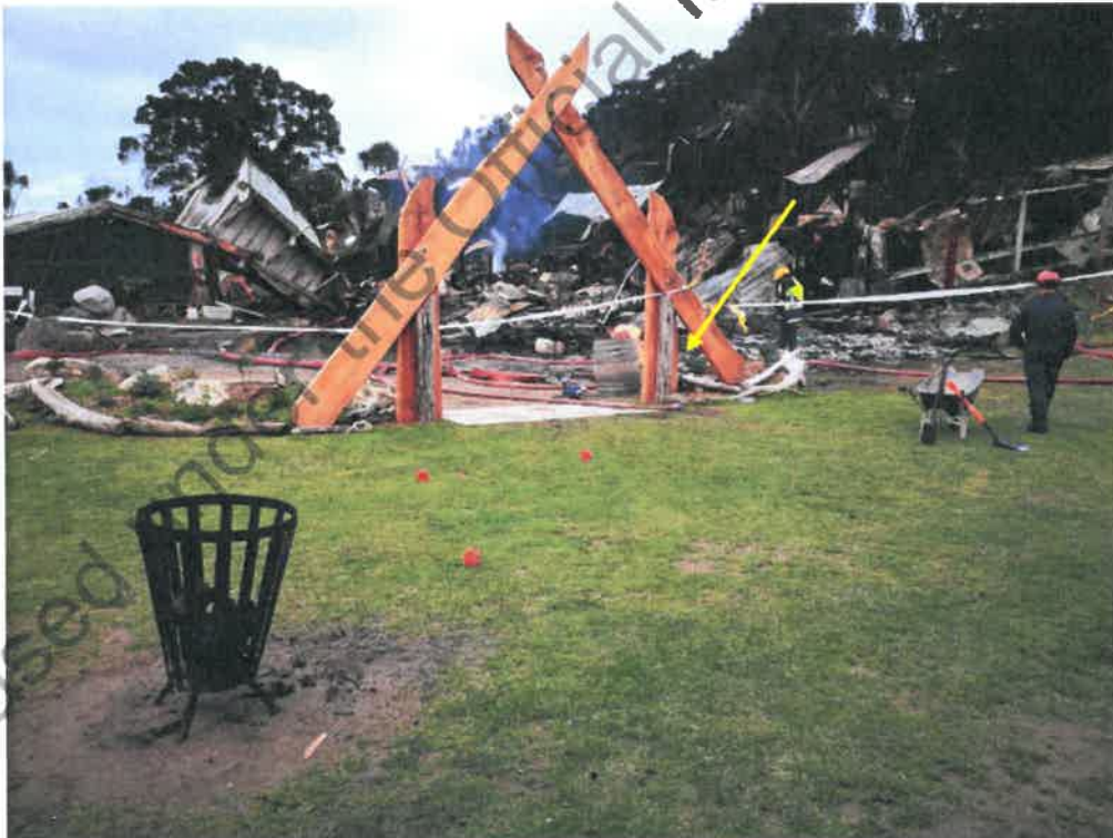
Photo 13 showing brazier location with embers spilled immediately on the northern side of the burner and orange markers showing location of further ember locations. The location of the storeroom wall believed to be point of origin of building fire is indicated by yellow arrow.
