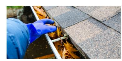
Figure 10: Example of debris accumulation in gutter
