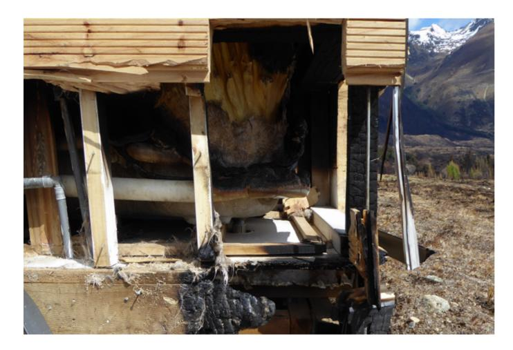
Figure 12: Example of how vulnerable timber cladding is to ember attack, radiant heat or direct flame. Fire has broken through and set bathroom inside alight. Öhau 2021 (Fire 3088958)
