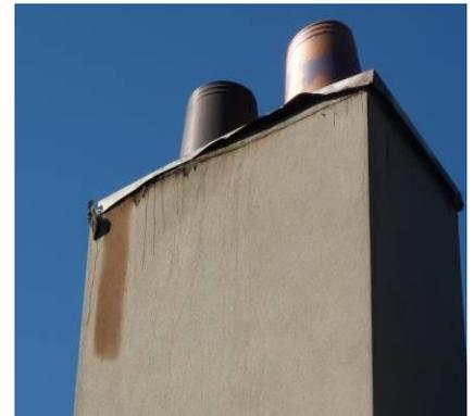
Fireplace manufacturers installation instructions require chimney chases to include construction aspects including adequate ventilation (top and bottom), specified clearances and importantly, non-combustible material to be used under the flashing.
