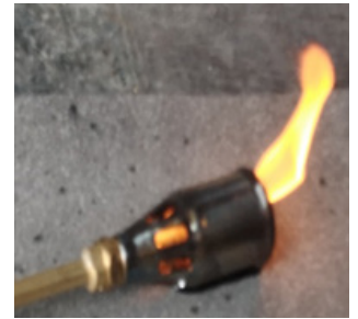
Hot works photos.
