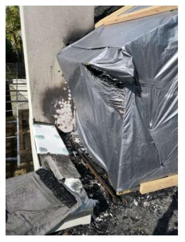
Photo 3 – shows damage to tarpaulin that had been used to protect the house after the initial fire.
