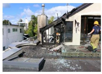
Photo 2: shows stainless steel capping which reflected sunlight onto timber cladding.
