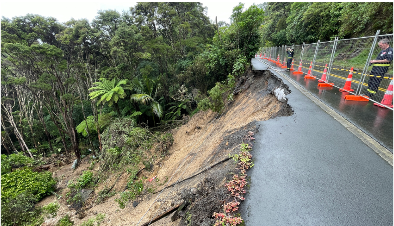
A major landslide in Titirangi, Auckland, covering the main access road, 29 January 2023. Courtesy of Dr Jan Kupec.
