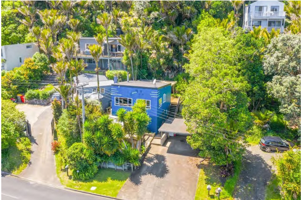
Figure 7 above. Firefighters were working at centre rear house before the landslide. CFO rescued a person from roof section of centre front house shown after the landslide in figure 8 below. (Real estate photo)
