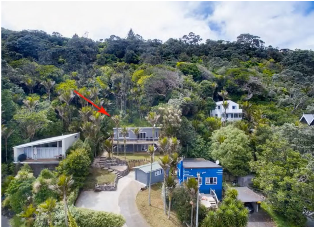
Figure 6 above. Firefighters were working at the centre house indicated by the arrow before the landslide. (Real estate photo)
