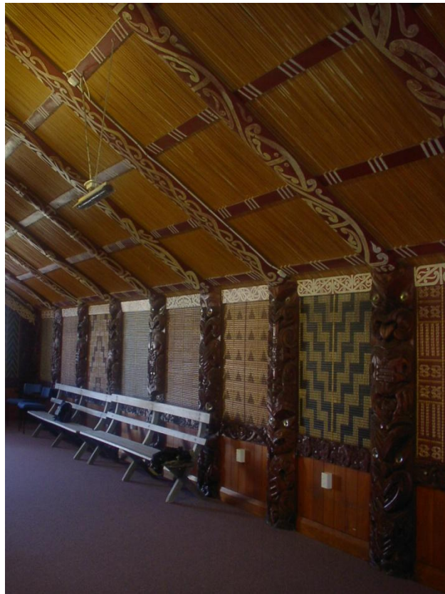
Figure 13: Toetoe kakaho on ceiling (Duncan et al, 2004)
