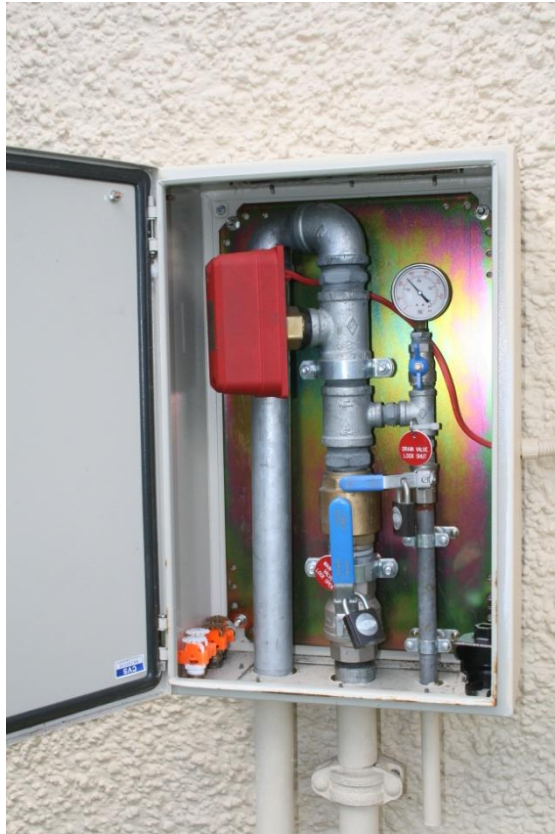
Figure 19: Domestic valveset
