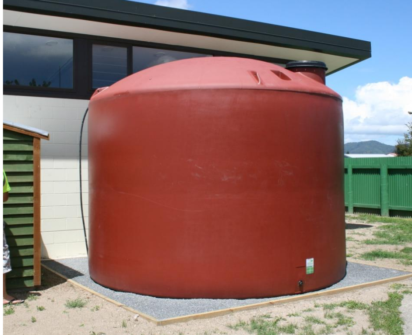
Figure 18: Plastic storage tank – 30,000 L
