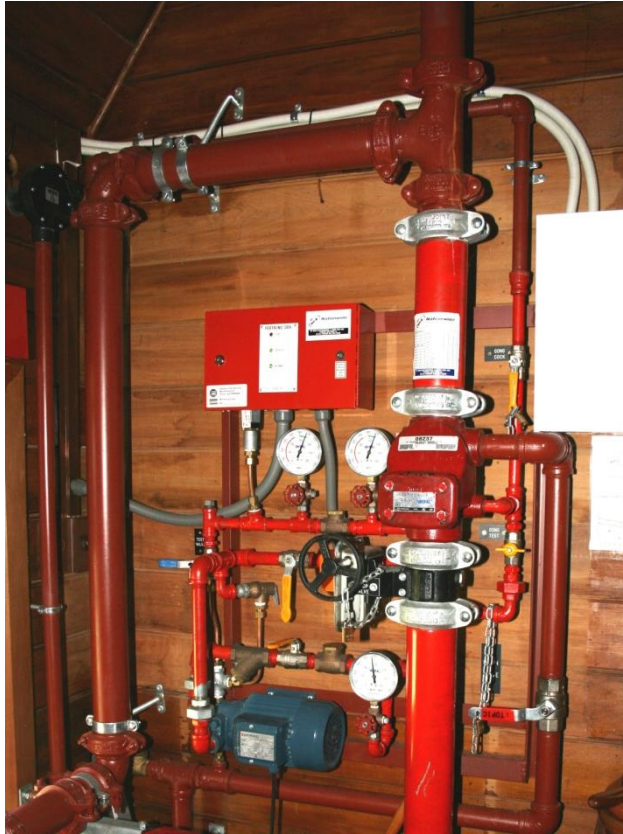
Figure 21: NZS 4541 OH1 valveset
