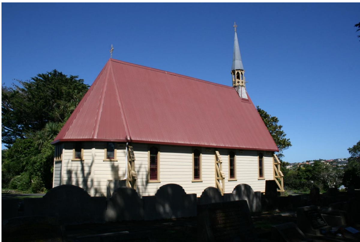
Figure 4: St Alban's Church, Pauatahanui, Porirua
