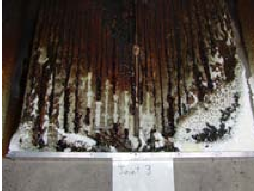
Figure 4.52: Remaining EPS core in lower portion of joint 3 panel.
