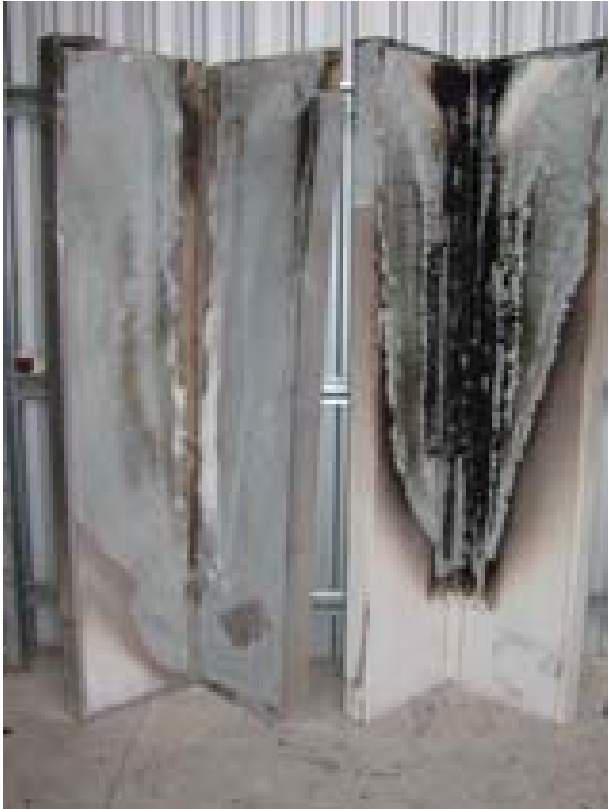
Figure 4.49: Corner joint specimens, fire exposed side, trials 4 to 5 from left to right.
