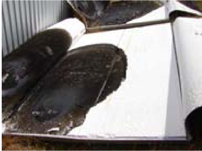
Figure 4.31: Remaining EPS core in trial 1.
