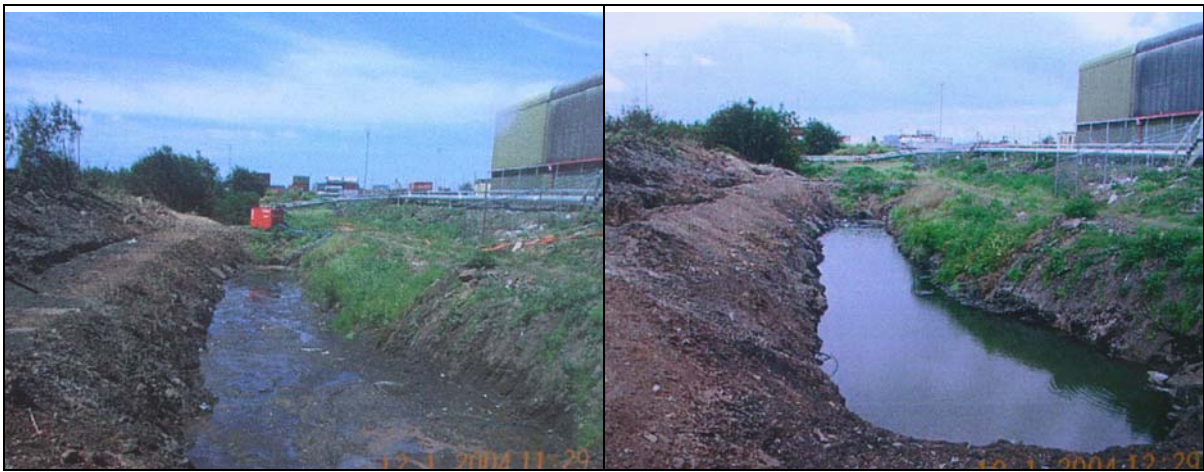
Figure 16: Carter Holt Harvey Pulp & Paper stormwater ponds, after the December 2003 fire. Left: Pond filled with decomposing paper, 12 January. Right: Pond after paper sludge removed, 19 January. (Photos: Auckland Regional Council).
