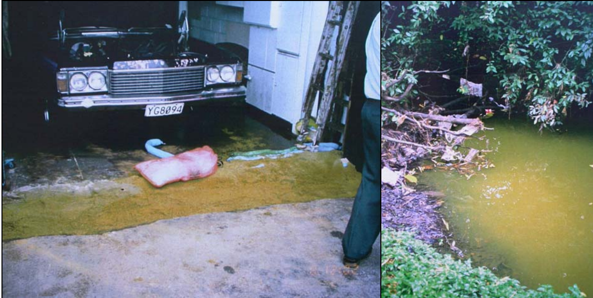
Figure 21: Otahuhu Chromeplaters Ltd, 7 – 8 May 2000. Left: Sand used as a bund and to absorb chromic acid displaced from acid baths by fire-water. Right: Stream coloured yellow by chromic acid due to the fire-water discharge (before sand bunding). (Photos: Auckland Regional Council).
