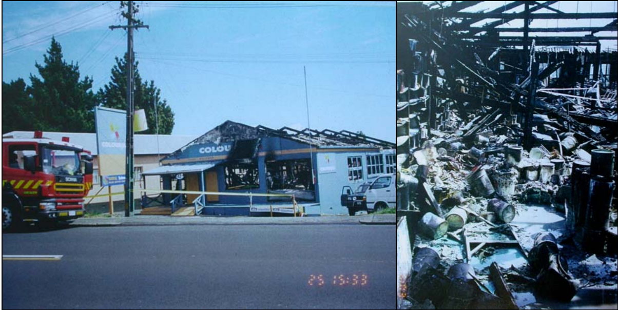
Figure 19: Colourplus paint manufacturers, Mt Roskill, 24 – 25 Jan 2002. Left: Paint manufacturing building damaged by fire. Right: Interior of building showing spilt paint likely to be flushed by fire-water. (Photos: Auckland Regional Council).
