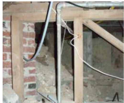
Figure 0-4 Structural Connection likely to move apart in an Earthquake Figure 0-5 Pipe work interweaving within the Structure
