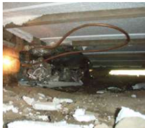
Figure 0-6 Gas Pipe work laid on the Ground under Dwelling Figure 0-7 Copper Gas reticulation with reserve flexibility of tubing
