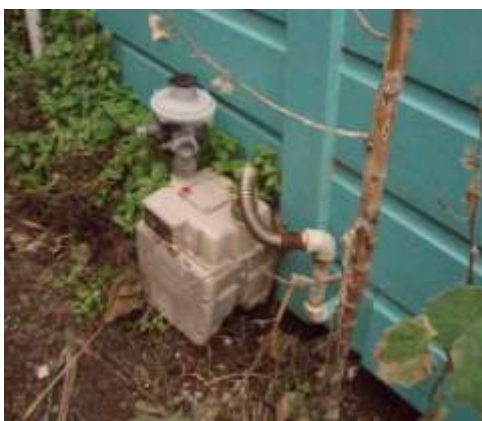
Figure 0-2 Flexible Gas Connection into Sub-floor Wall
