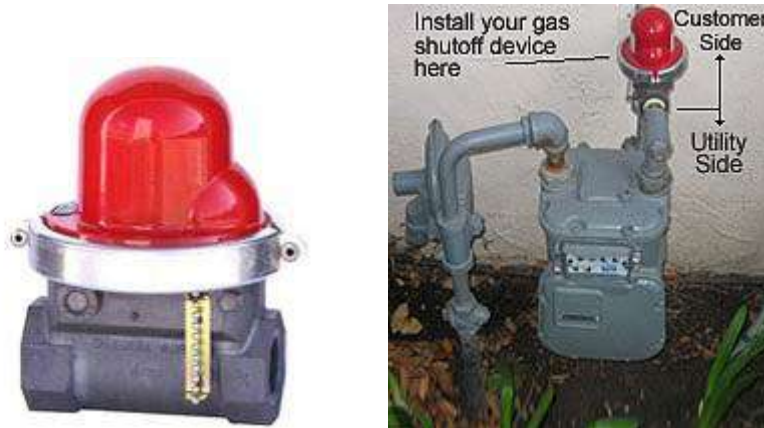
Figure C1 Koso brand Seismic Shutoff Valve (Source: BRANZ 2000; Earthquake Store.com 2007)
