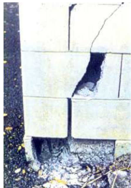
Figure 0-8 Wall separating from Exterior Foundation wall (Source: BRANZ 2003)
