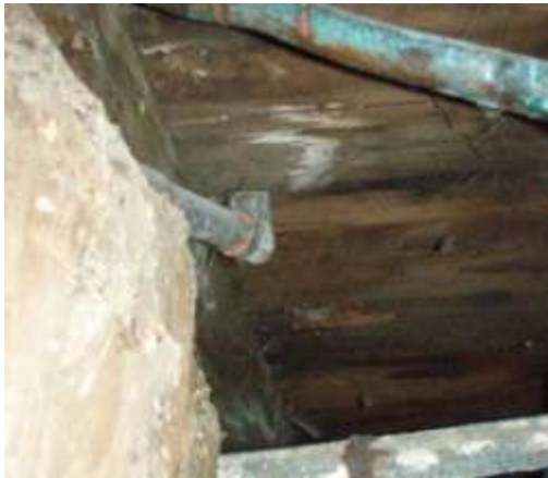
Figure 0-8 Rigid Gas Connection into Flooring of dwelling Figure 0-9 Flexible Gas Connection into Gas Appliance
