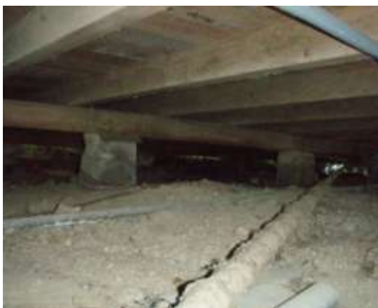
Figure 0-6 Gas Pipe work laid on the Ground under Dwelling Figure 0-7 Copper Gas reticulation with reserve flexibility of tubing
