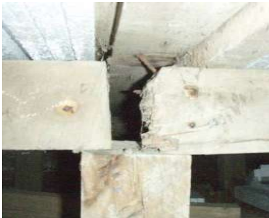
Figure 0-4 Structural Connection likely to move apart in an Earthquake Figure 0-5 Pipe work interweaving within the Structure
