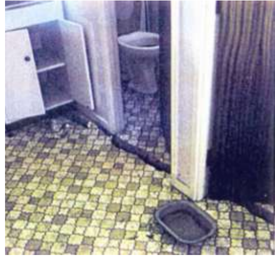
Figure 0-11 Slab on Ground showing relative sliding difference between the Dwelling and Ground; note the prior location of Services (Source: BRANZ 2003)
