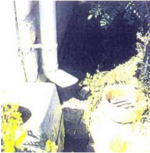
Figure 0-11 Slab on Ground showing relative sliding difference between the Dwelling and Ground; note the prior location of Services (Source: BRANZ 2003)
