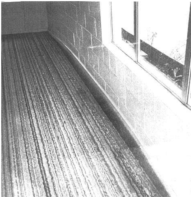
Figure 0-8 Wall separating from Exterior Foundation wall (Source: BRANZ 2003)
