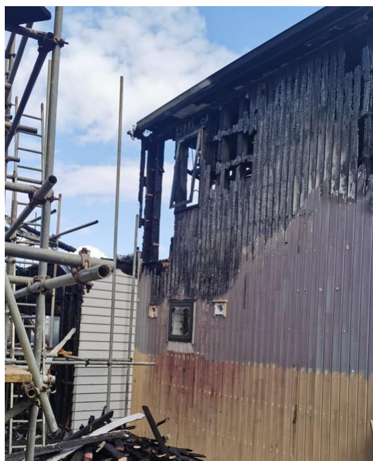
Figure 9: Partial northern external wall of Dwelling 2 – View from Dwelling 3
